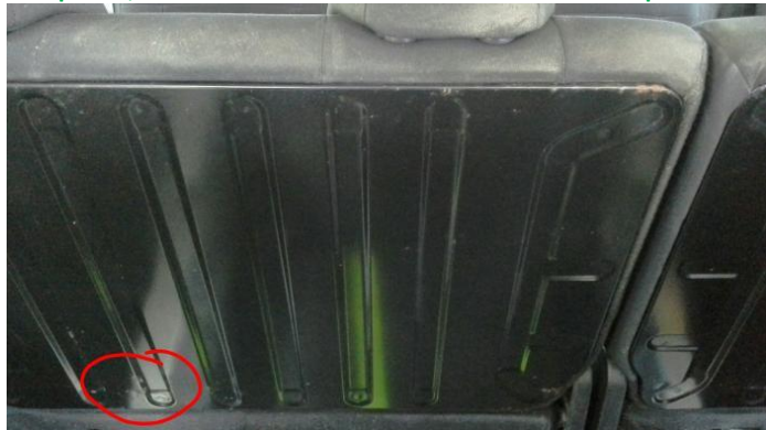
Acceptable, minor dents and scratches to metal seat back panel
